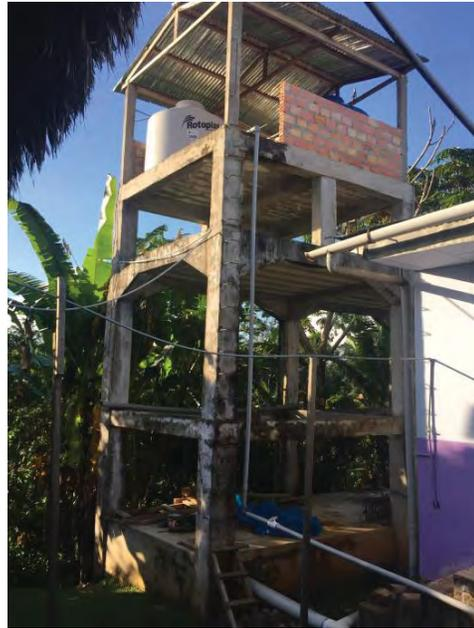
Fig. 1. Water tower in Nauta, Peru. Fiberglass tanks can be seen at the top, and the main transmission line can be seen exiting the bottom right of the photo.
