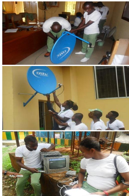
Figure-6: Installing and Tracking Satellite Broadcast Signals
