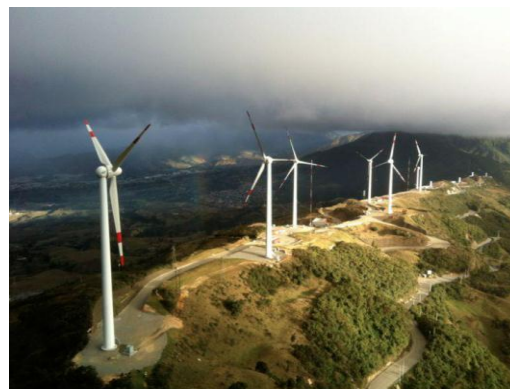
Fig. 1.- Panoramic view of the Villonaco Wind Power Plant.
